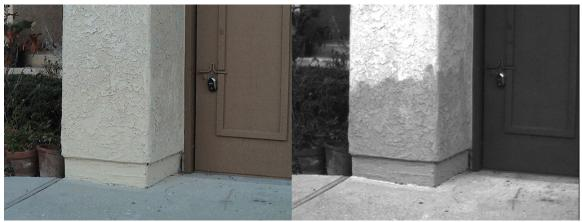
Figure 9. Freshly repainted stucco exterior wall. The fresh paint is dark in appearance. Left – color, right – near-UV
