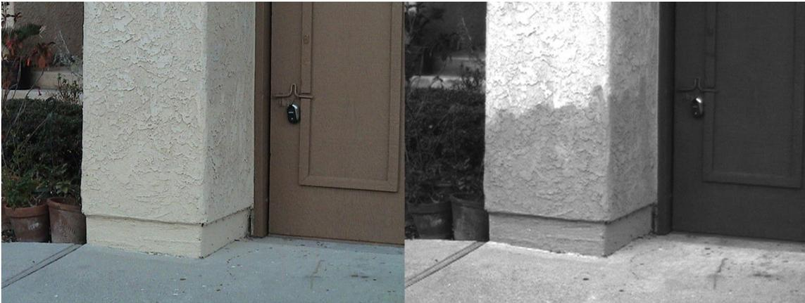
**Figure 9. Freshly repainted stucco exterior wall. The fresh paint is dark in appearance. Left – color, right – near-UV**
