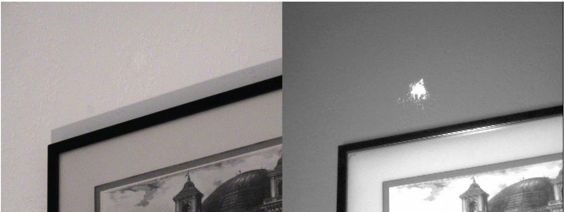
**Figure 13. Spackle on walls painted with white latex paint. Left – color, right – near-UV**
